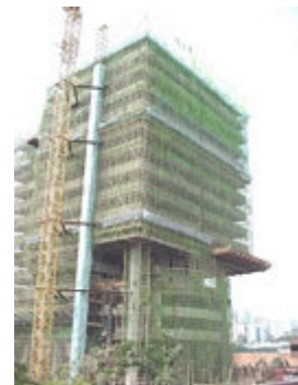
Fig. 1.1 Typical bamboo scaffold - Double Layered Bamboo Scaffold (DLBS)
